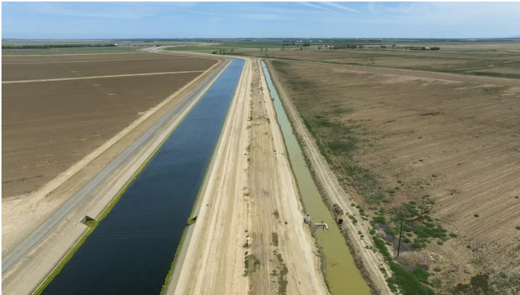
The Central Valley Project includes the Delta-Mendota Canal, left, in Firebaugh. (Brian van der Brug / Los Angeles Times)
